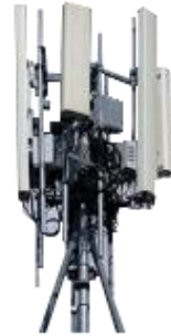
5G Base Station
